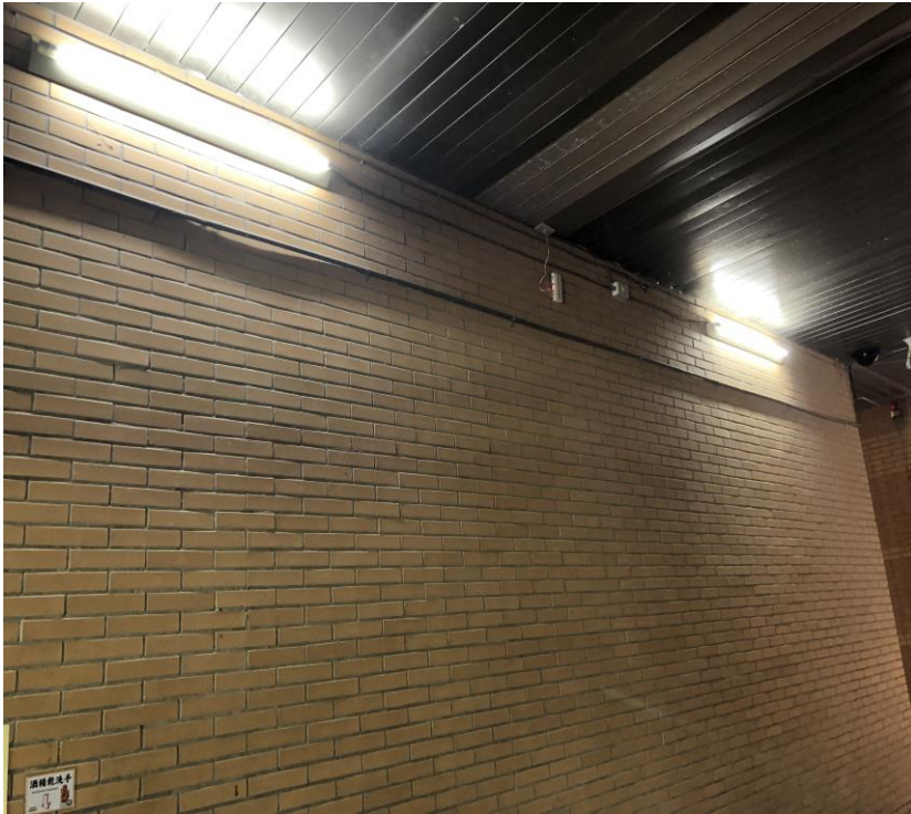
捲揚電梯走廊燈具更改
