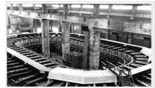
Uranium for "Little Boy" was enriched in calutrons and by gaseous diffusion at Oak Ridge, Tennessee.
